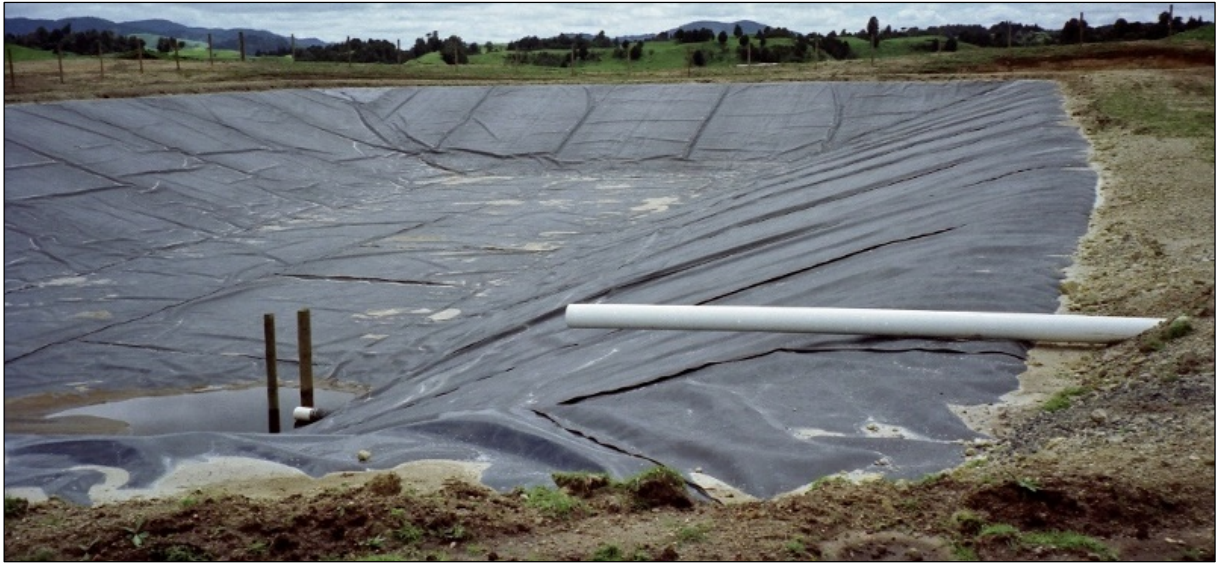
Figure 9 Anaerobic pond, installed in 1999.
