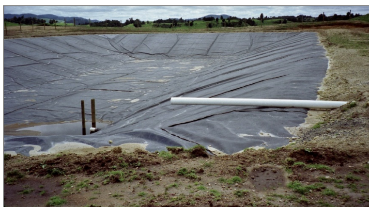
Figure 2 Wastewater storage pond, installed in 1999.
