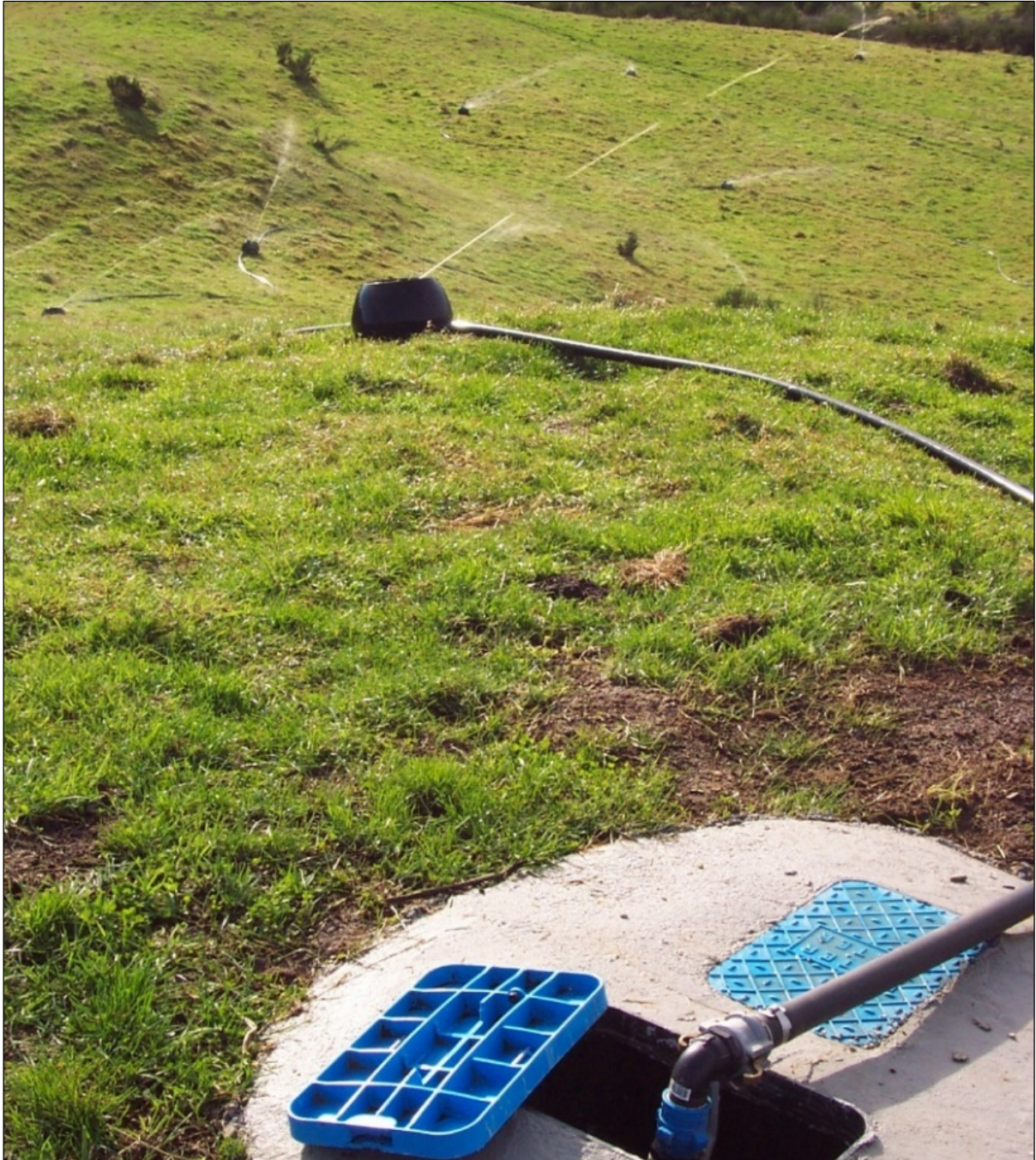
Figure 12 K-Line irrigation system.
