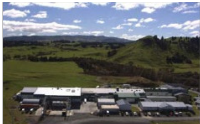
Figure 1 Crusader Meats plant
